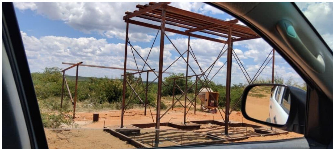
The water tank stands being constructed at the capped borehole
